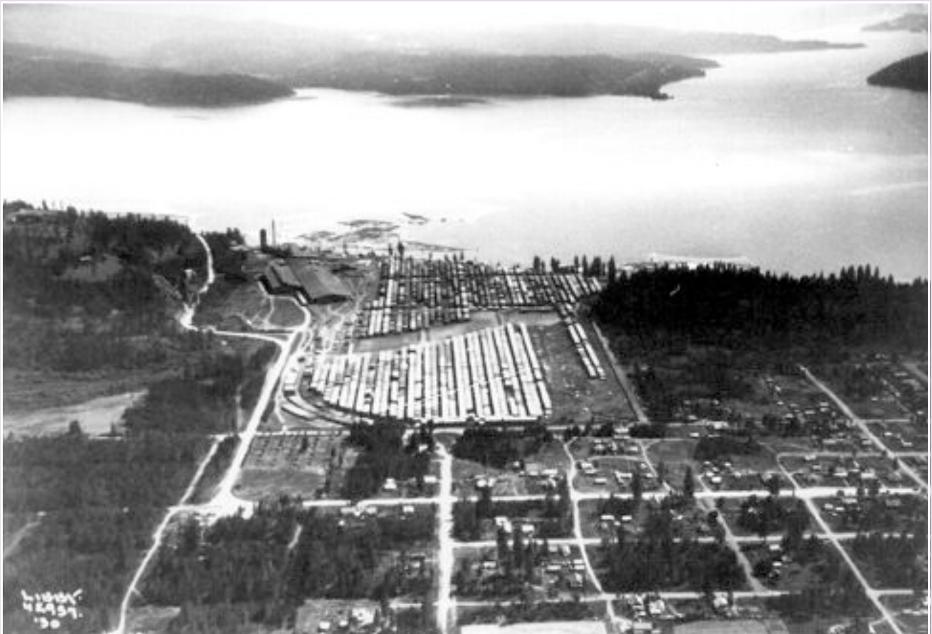
Potlatch Rutledge Mill, Coeur d'Alene, July 1930. The mill site is now a golf course. [Libby Studio, courtesy Spokane Public Library]
