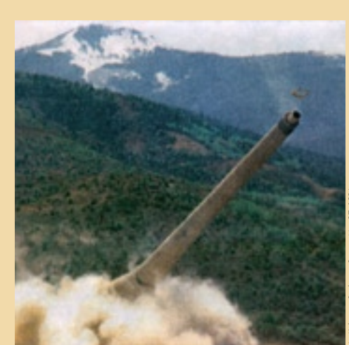
Blowing up the 715-foot-tall smoke stack at the Bunker Hill lead smelter, May 26, 1996. The once-dormant mountainsides are beginning to recover.
