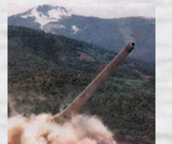
Blowing up the 715-foot-tall smoke stack at the Bunker Hill lead smelter, May 26, 1996. The once-dreaded mountainsides are beginning to recover. photo: Liz Kishimoto, Spokesman-Review , May 27, 1996
