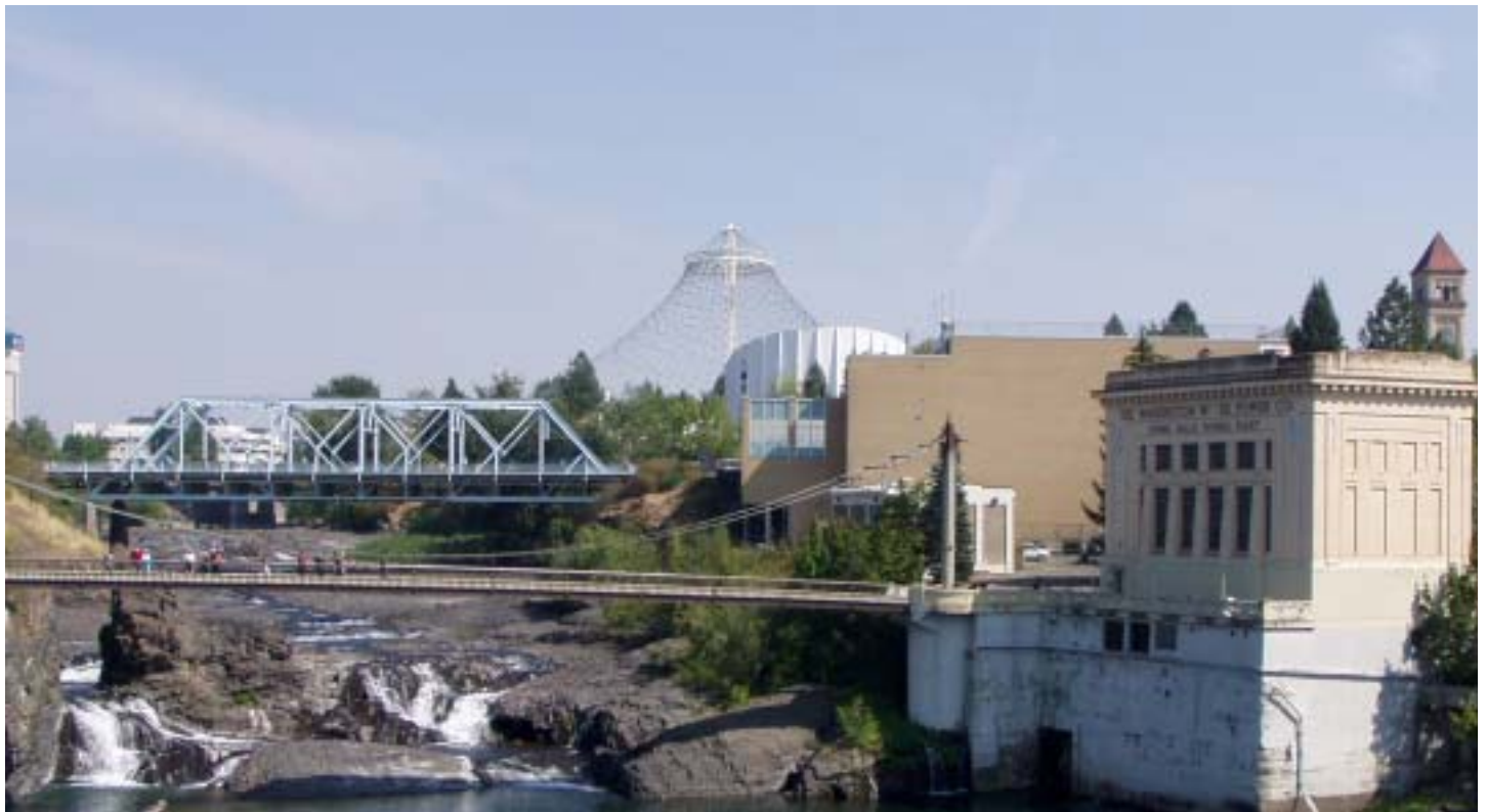
(8) Avista (Washington Water Power). Avista's dams in the early 1900s extirpated the river's once-prized salmon runs. Avista's PCBs pollute the river. The Post Falls Dam is dewatering the river. Avista's facilities in downtown Spokane divert water (what little there is) from Spokane Falls. And now Avista has applied for water rights in Idaho, pumping more water from the Aquifer and further damaging the Spokane River. Avista has done more to destroy the Spokane River than any other single institution. Will that ever change?
